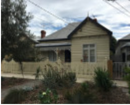
31 King Street FITZROY NORTH
