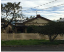
29 King Street FITZROY NORTH
