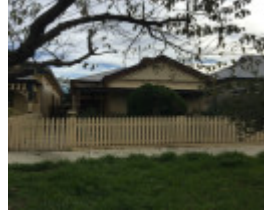
29 King Street FITZROY NORTH
