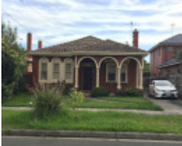
5 Lowan Street BRUNSWICK EAST
