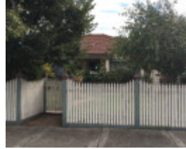
15 Lowan Street BRUNSWICK EAST
