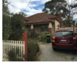
23 Lowan Street BRUNSWICK EAST
