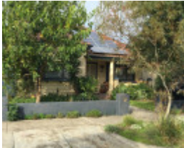
14 Lowan Street BRUNSWICK EAST
