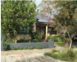
14 Lowan Street BRUNSWICK EAST
