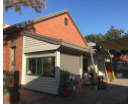
Rear elevation showing verandah addition.
