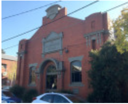
Grosvenor Street facade.
