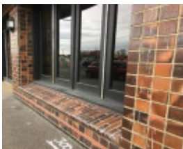
2017 1938 facade window opening.jpg
