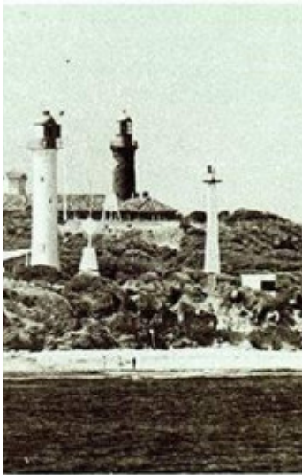
sive system of leading lights on tring the entrance to Port Phillip Ba hite Low lighthouse in line with the through the middle of the channel
