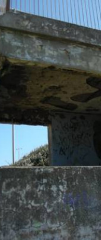
2018, World War II bunker on southern boundary.jpg
