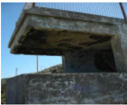
2018, World War II bunker on southern boundary.jpg
