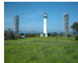
2018, Looking south-east_Murray tower on left_Hume Tower on right.jpg
