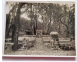
Chapel under construction
