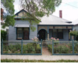
283 Myers St, Geelong East
