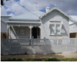
288 Myers St, Geelong East
