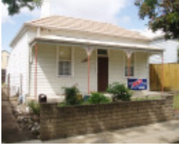
292 Myers St, Geelong East
