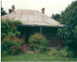
H01987 log cottage poowong front 2001
