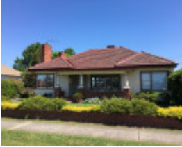
House, 23 Rogers Street
