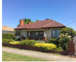
House, 23 Rogers Street
