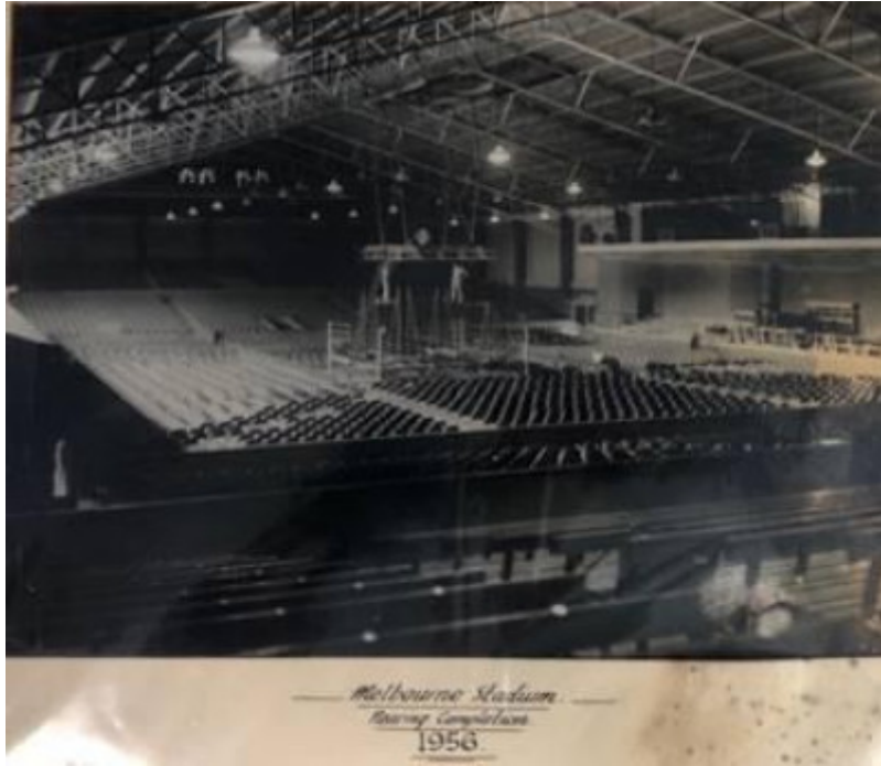
1956, interior nearing completion.jpg
