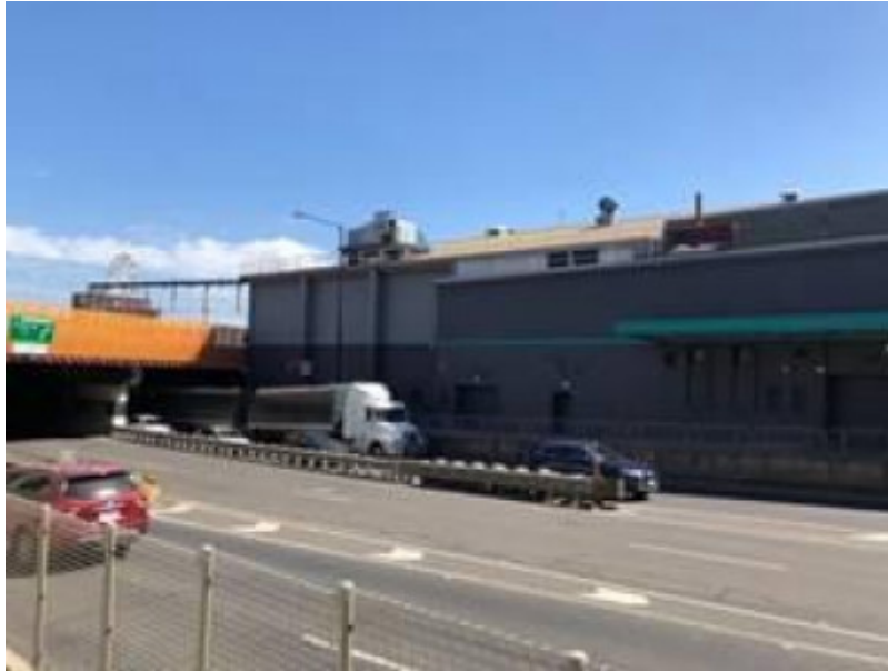
2018, Dudley Street from south-east.jpg
