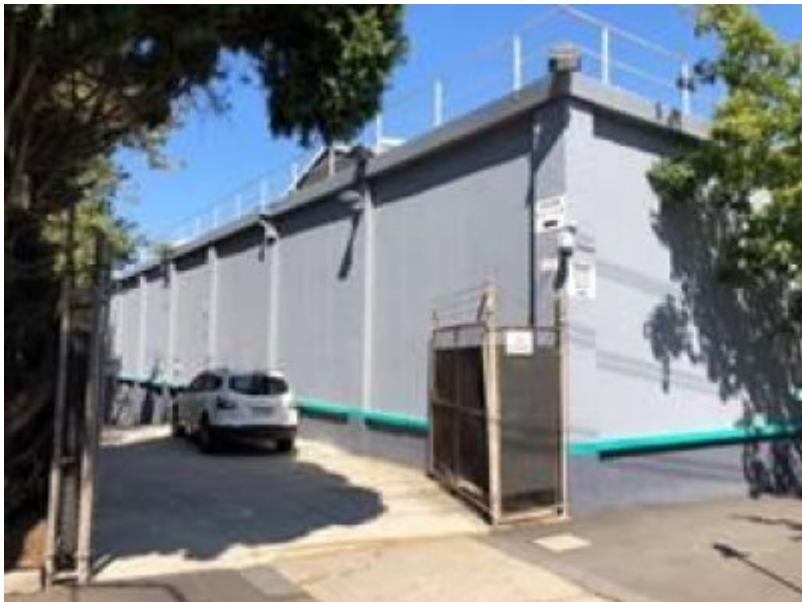
2018, east elevation from north east.jpg
