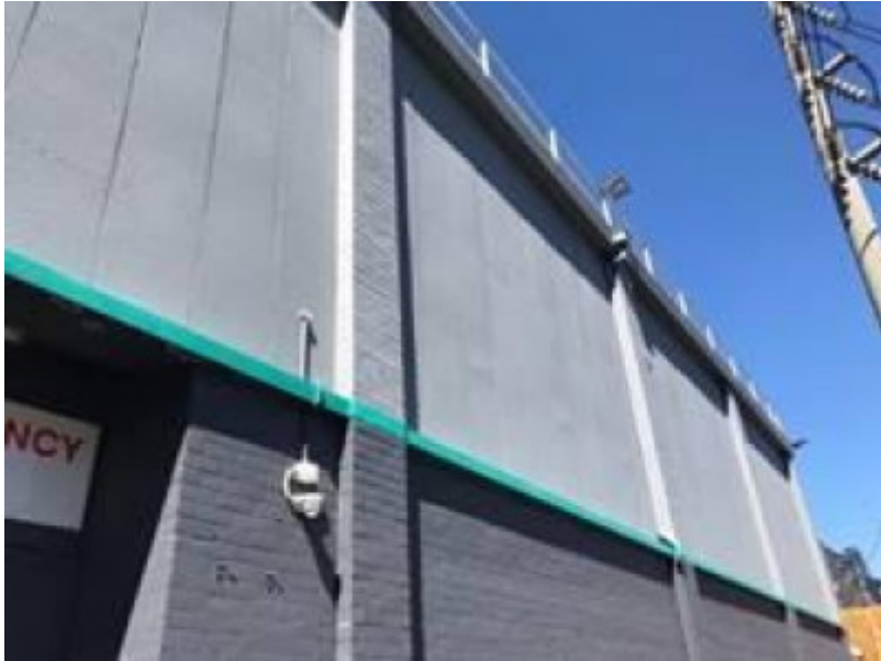
2018, details showing concrete panels.jpg
