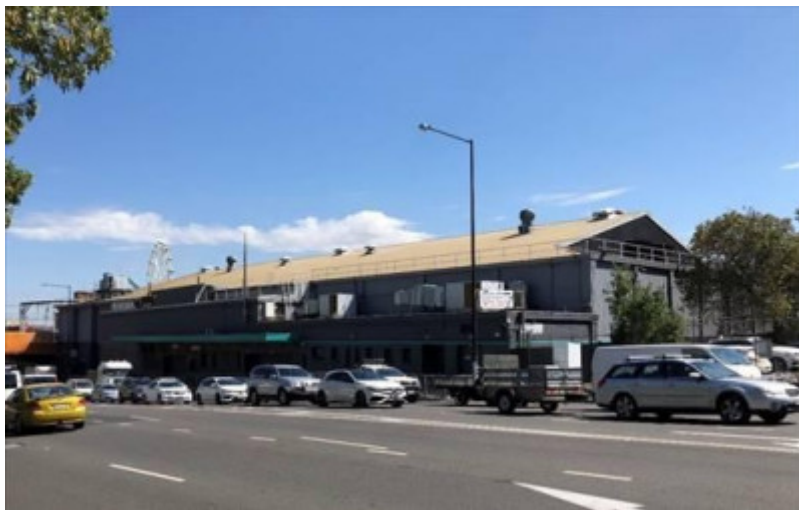
2018, Dudley Street elevation.jpg
