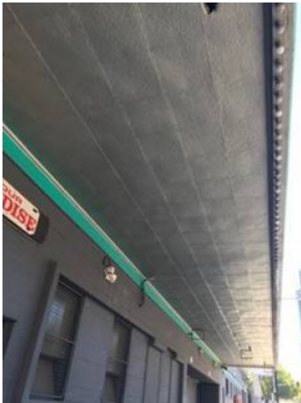
2018, underside of awning.jpg
