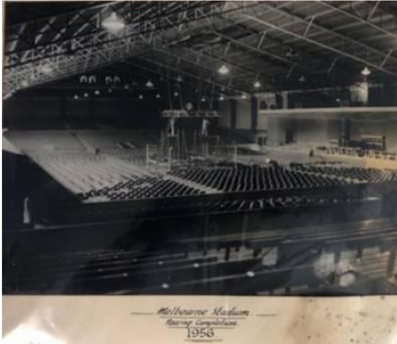
1956, interior nearing completion.jpg
