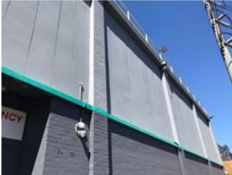
2018, details showing concrete panels.jpg
