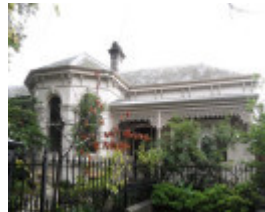
3 and 5 Avondale Road Figure 4 Front facade of 5 Avondale Road. Note casement box bay window beneath verandah. (Source: Context, 2017).jpg
