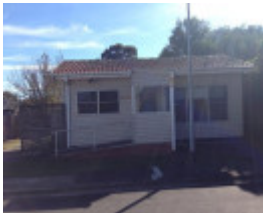
St James' Estate - former community meeting room converted to residence (no.18)
