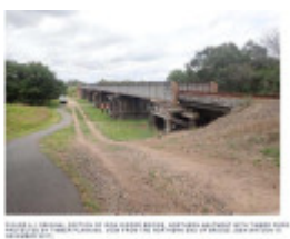
2017, Northern approach, 1888 section .jpg
