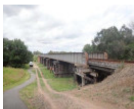
2017, northern approach 1888 section.jpg
