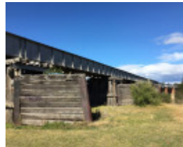
2018, Timber cutwaters and piers.jpg
