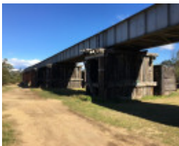
2018 timber piers 1888 section.jpg
