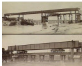
1896 Girders being moved into place with trolleys.jpg
