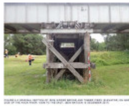
2017, 1888 section, timber piers and iron girders above.jpg
