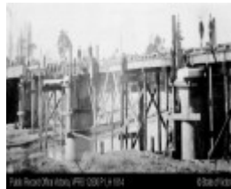
1896 Construction of masonry piers.jpg
