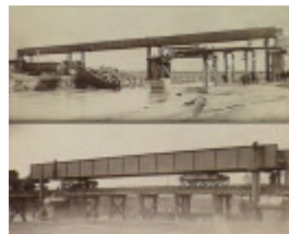
1896 Girders being moved into place with trolleys.jpg
