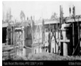
1896 Construction of masonry piers.jpg
