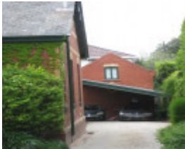
32 Sutherland Road Armadale - coach house
