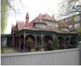
29 Denbigh Road Armadale
