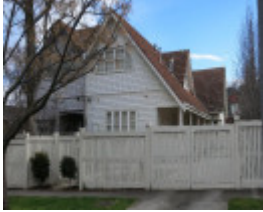
5 & 7 Tollington Avenue Malvern East
