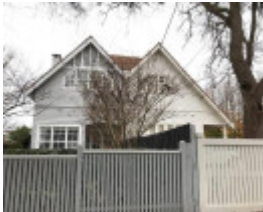
5-7 Tollington Avenue, Malvern East
