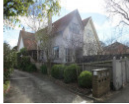
5 & 7 Tollington Avenue Malvern East
