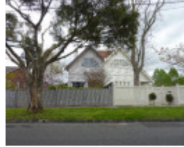
5 & 7 Tollington Avenue Malvern East
