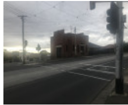
Brunswick West Tramway Substation
