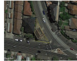
Brunswick West Tramway Substation from above
