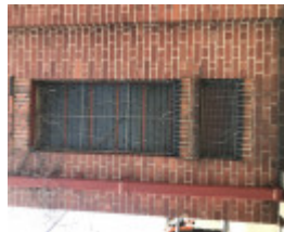
Tapestry brick and window grill
