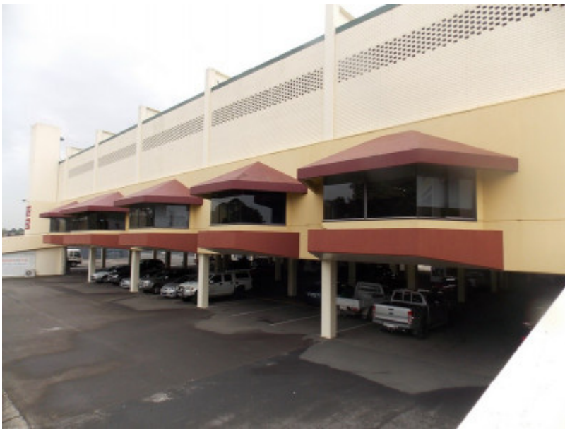
General view of the 1976 additions from west (carpark side), looking north-east.jpg
