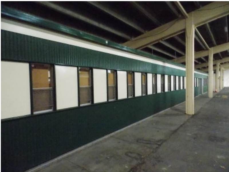
Original tote building in undercroft area north end showing hatch-like windows.jpg
