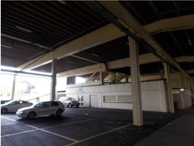
General view of undercroft area showing exposed structure and low-rise infill.jpg
