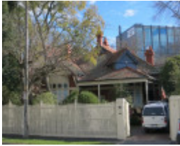
5 Burke Road Malvern East
