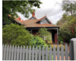
5 Burke Road, Malvern East
