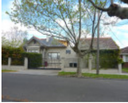
1121 Dandenong Road Malvern East
