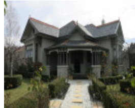
1121 Dandenong Road Malvern East
