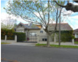
1121 Dandenong Road Malvern East
