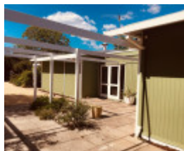
West courtyard looking north east
