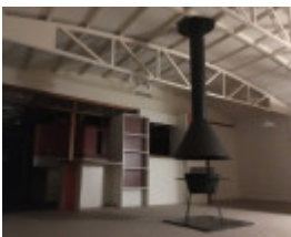
Looking south west from living room
