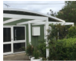
North courtyard towards entry
