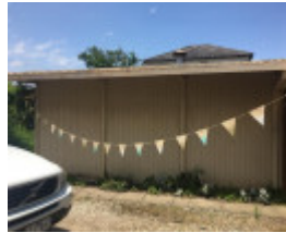
Grant House 2018, West facing elevation (rear module).jpg
