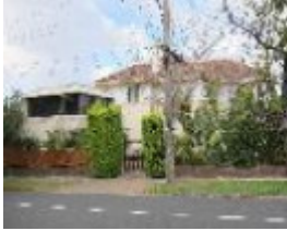
486 Burke Road, seen from Pine Avenue.
