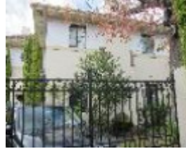
486 Burke Road, seen from Pine Avenue.
