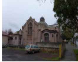
Canterbury Road, 146 CANTERBURY PRESBYTERIAN CHURCH rear
