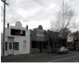
Canterbury Road, 351-359 VICTORIAN SHOPS
