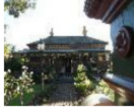
Chatham Road, 35 KAIAPOI front
