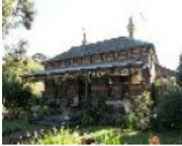
35 Chatham Road, Canterbury KAIAPOI
