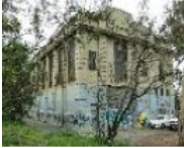
Myrtle Road Warburton Road, 26A & 2B EAST CAMBERWELL SUBSTATION
