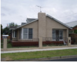
382 Myers St, Geelong East
