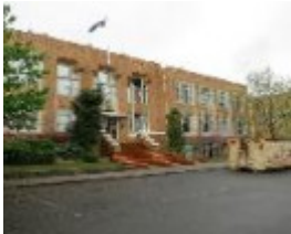
Prospect Hill Road, 100a CAMBERWELL HIGH SCHOOL
