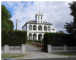
Aberfeldie Street and Waverley Street Precinct
