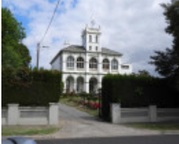
Aberfeldie Street and Waverley Street Precinct
