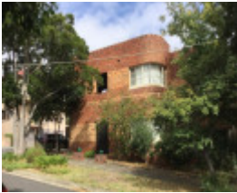
2 Denmark Hill Road.jpg
