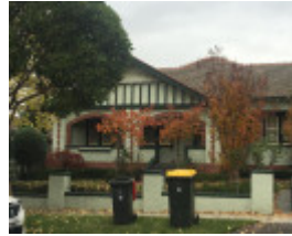
23 Ballater Street Essendon
