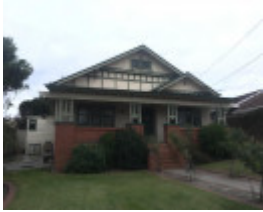
25 Ballater Street Essendon
