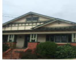
25 Ballater Street Essendon
