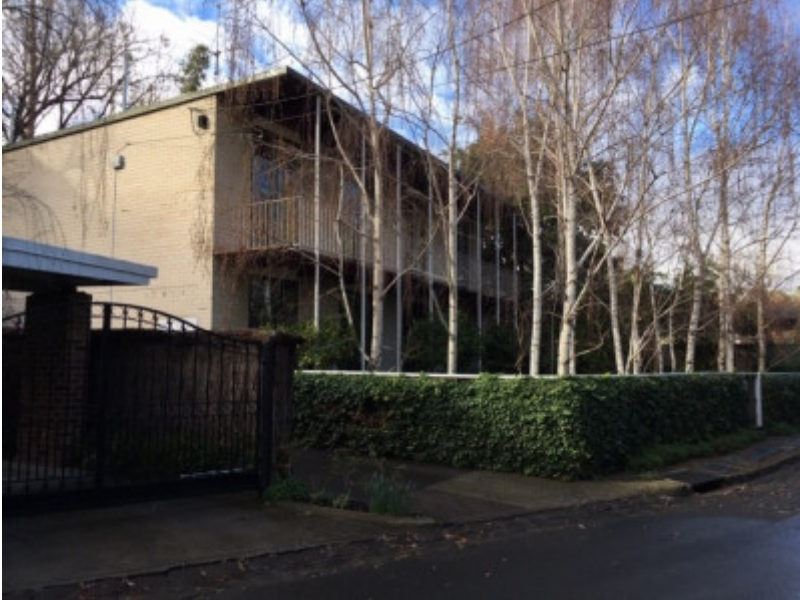
Brett House exterior.jpg
