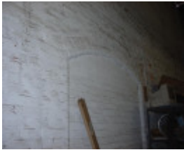
Segmental arched opening in south wall
