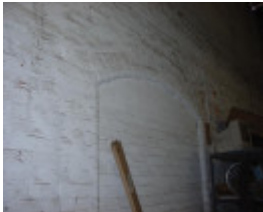
Segmental arched opening in south wall
