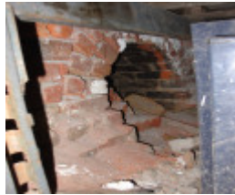
View of flue entrance on south side of chimney
