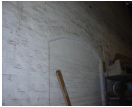
Segmental arched opening in south wall
