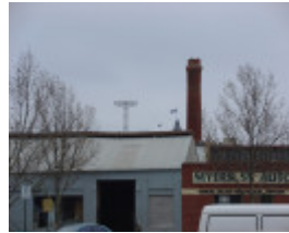
View of chimney from across Myers Street
