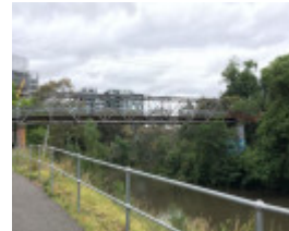
Walmer Street Bridge - 2019
