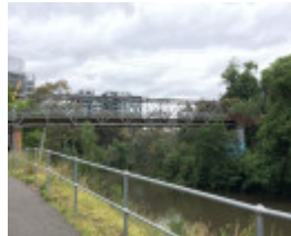
Walmer Street Bridge - 2019
