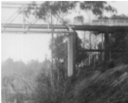
Walmer Street Bridge - c1920s
