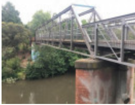
Walmer Street Bridge - view from south bank - 2019
