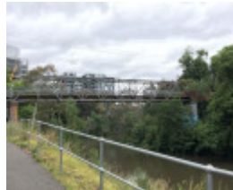
Walmer Street Bridge - 2019
