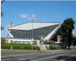
OLYMPIC SWIMMING STADIUM SOHE 2008
