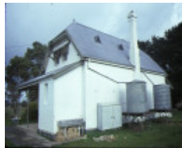
former primary school no688 cardigan rear view aug1984
