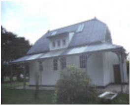
1 former primary school no688 cardigan front view aug1984
