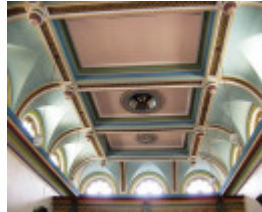
H2180 Clunes Town Hall - Hall ceiling 023
