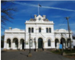
H2180 Clunes Town Hall & Court House
