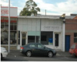
29 a Ryrie Street, Geelong
