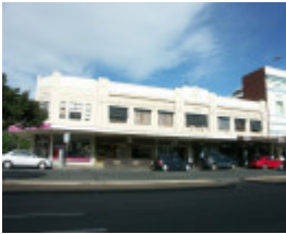
206 Ryrie Street, Geelong - Shops.JPG
