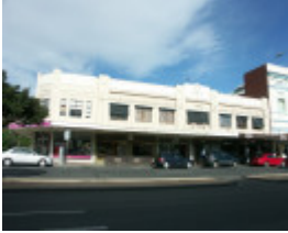
206 Ryrie Street, Geelong - Shops.JPG
