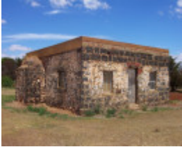
Cottage at Former Fulham Park
