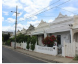
View along terrace row
