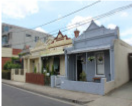
View along terrace row
