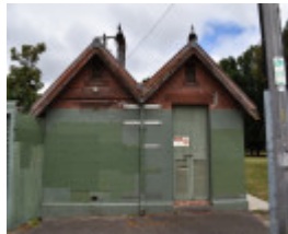
7 Methven Street, Brunswick East
